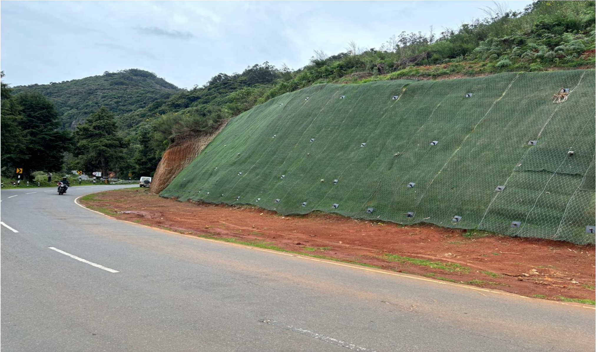
INSTALLATION OF THREE DIMENSIONAL EROSION CONTROL MAT
