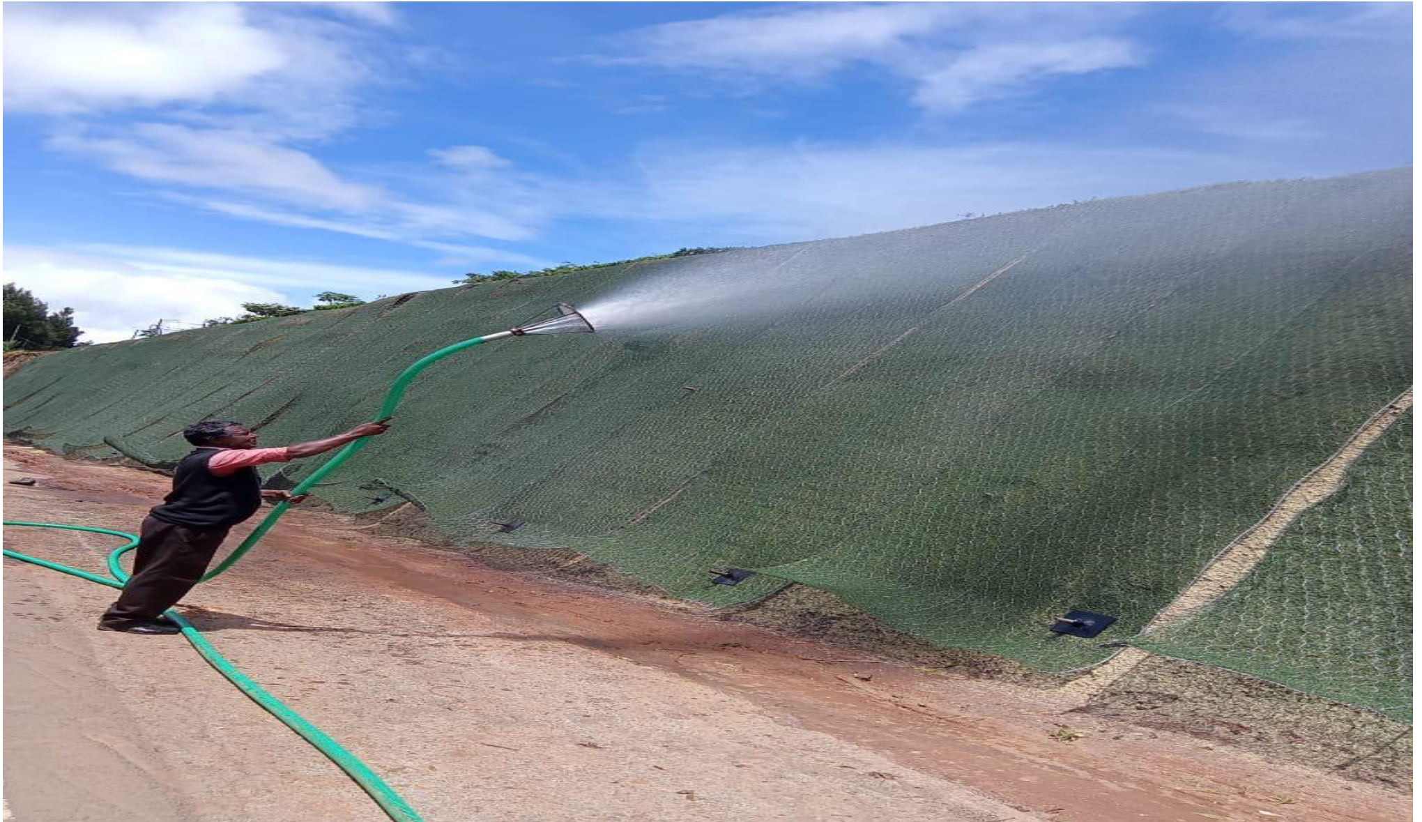
Maintenance (Watering) of Applied Surface
