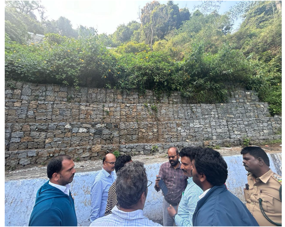
Photos: Gabion wall proved very effective in controlling soil erosion and land slides
