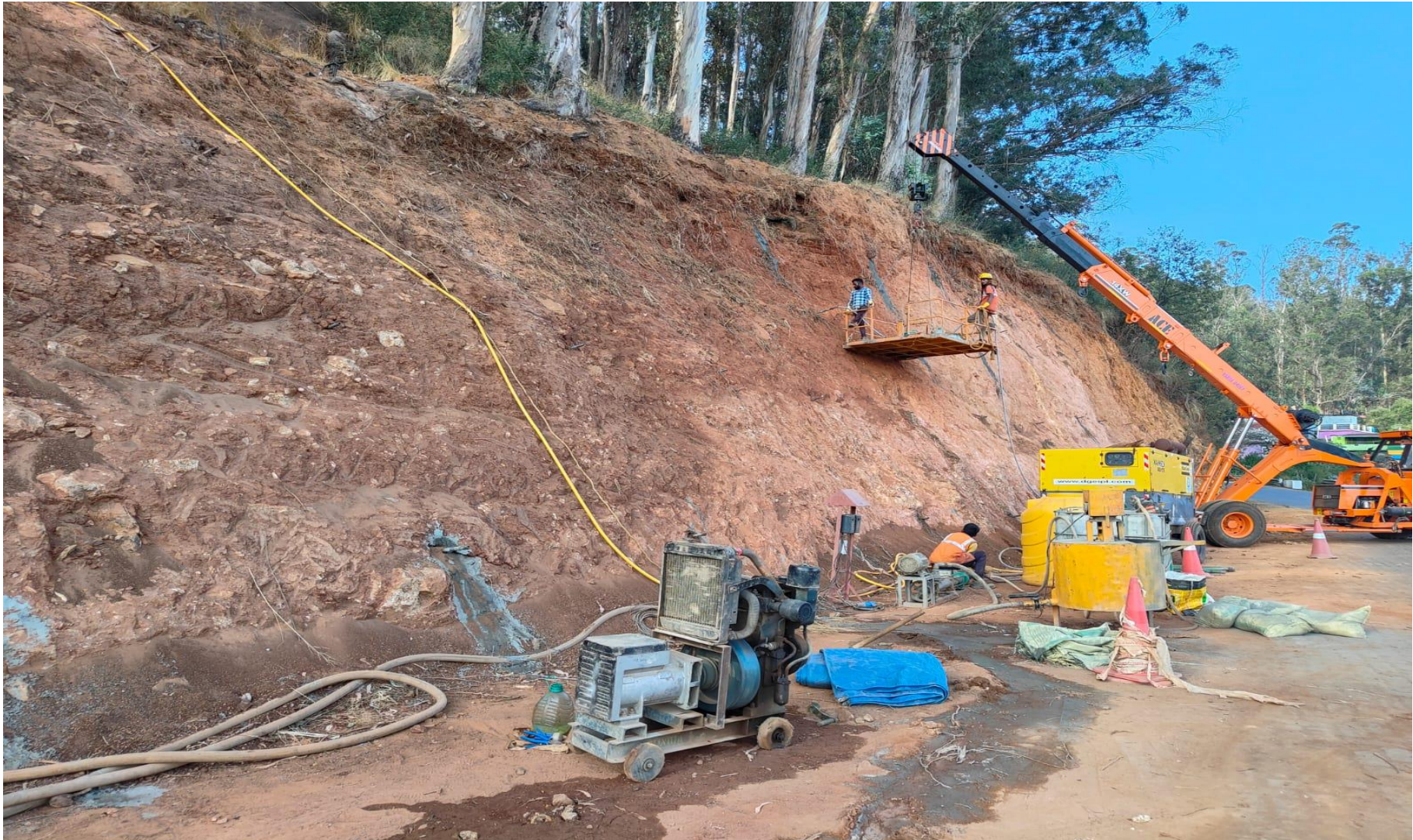
GROUTING WORK AT KM 1/6
