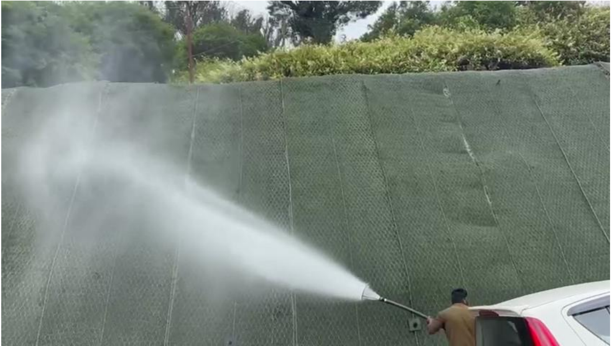
MAINTENANCE (WATERING) OF APPLIED SURFACE
