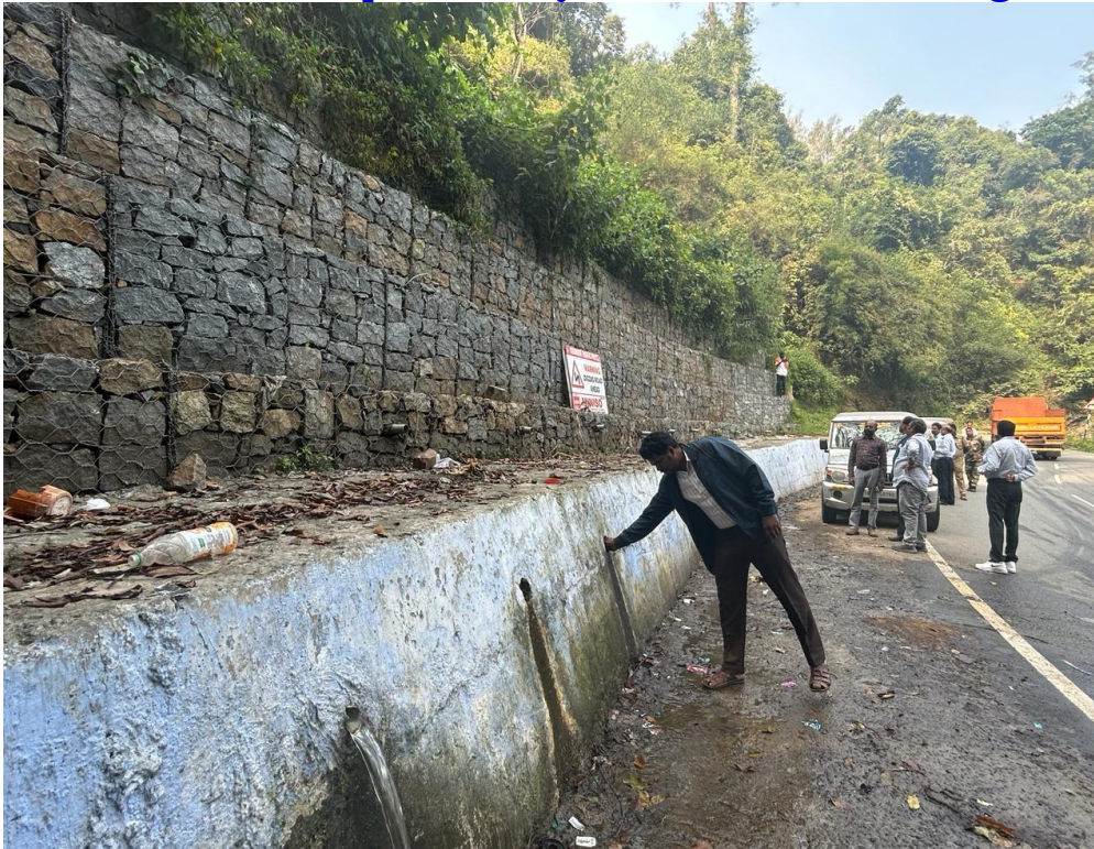
Photos: Gabion wall proved very effective in controlling soil erosion and land slides
