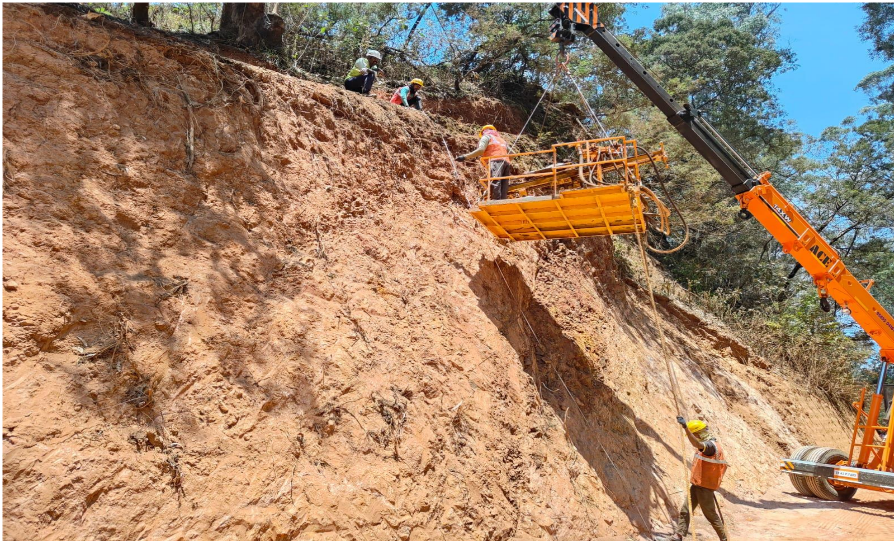
NAIL POSITION MARKING AT KM 0/8
